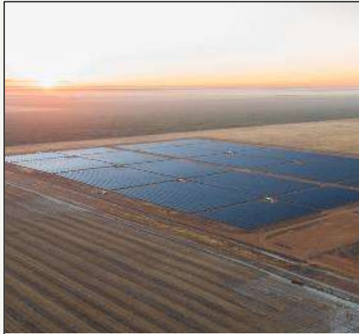
Greenough River Solar Farm Greenough River, WA (40.0 MWdc) Operational: Fully Contracted with Synergy (WA Govt owned retailer)
