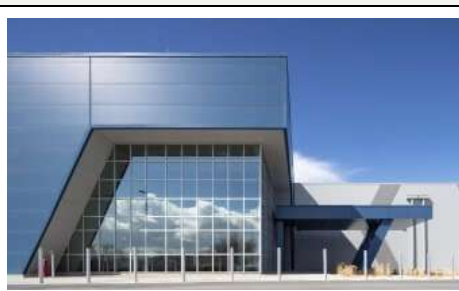
Aligned Data Centres
