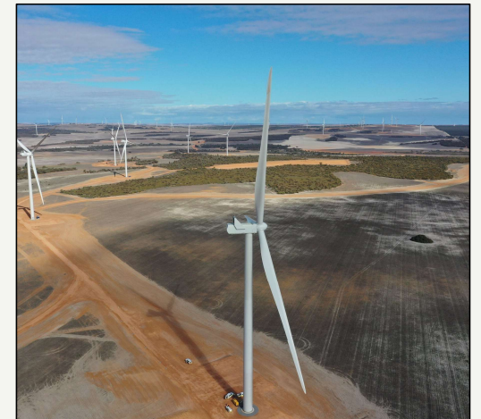
Warradarge Wind Farm Warradarge, WA (183.0 MWdc) Operational: Fully Contracted with Synergy (WA Govt owned retailer)
