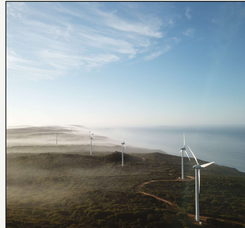
Albany & Grasmere Wind Farms Albany, WA (35.0 MWdc) Operational: Fully Contracted with Synergy (WA Govt owned retailer)
